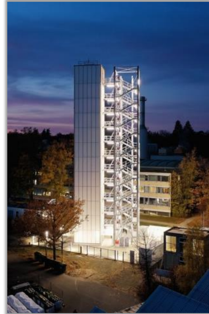
An Adaptive High-Rise Building
